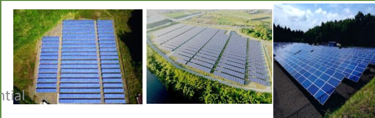
Kagoshima Total 15 MW COD 2014 ~ 2018 Under construction
