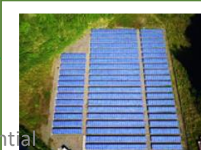
Kagoshima Total 15 MW COD 2014 ~ 2018 Under construction
