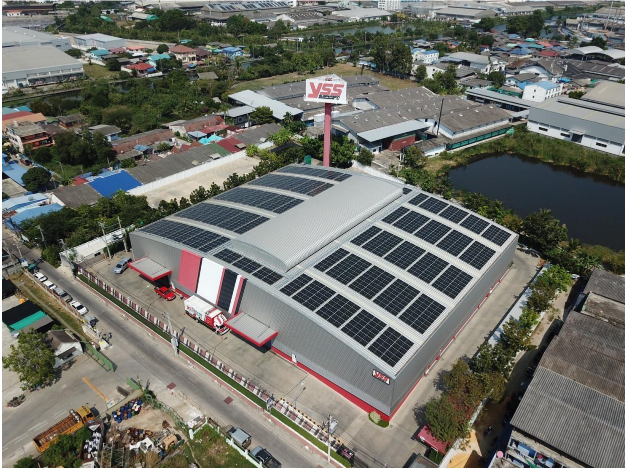
Solar Rooftop Project
